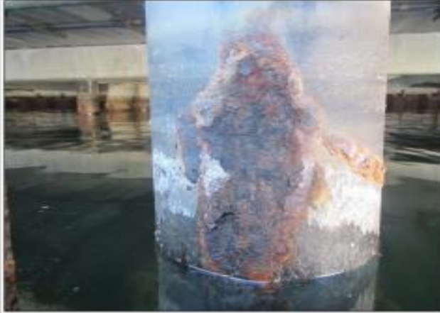
Docks 3 and 4 current condition
